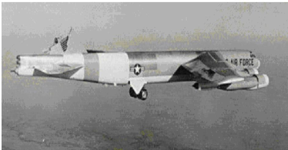
*Fig. 1. During a test flight, the vertical stabilizer of the B-52H, flying at a height of about 5 000 feet above New Mexico, is cut off in the event of large overloads. Six hours later, the crew managed to make the first and only B-52 landing without a vertical stabilizer [6].*
